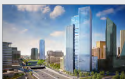
FIELD STREET TOWER Dallas CBD 529,038 RBA 529,038 Max Avail. SF Withheld Rents Hillwood Development
