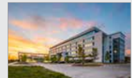
FOURTEEN555 - PHASE II Far North Dallas/Lower Tollway 239,909 RBA 239,909 Max Avail. SF Withheld Rents Cawley Partners
