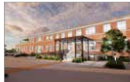
ARMOUR BUILDING North Fort Worth 57,254 RBA 26,839 Max Avail. SF 53.1% Leased Withheld Rents U.S. Energy
